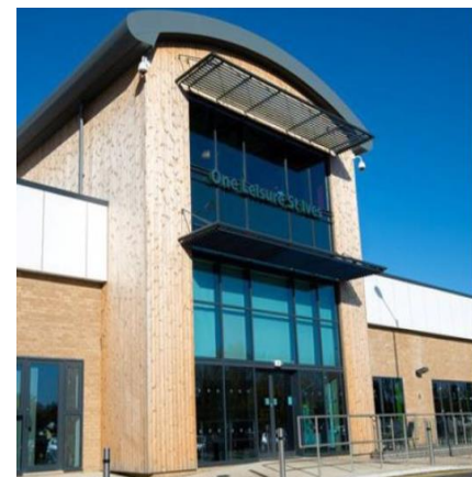
A view of the One Leisure St Ives Centre
