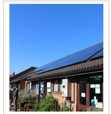
*The school's solar PV array on the south-facing roof.*
